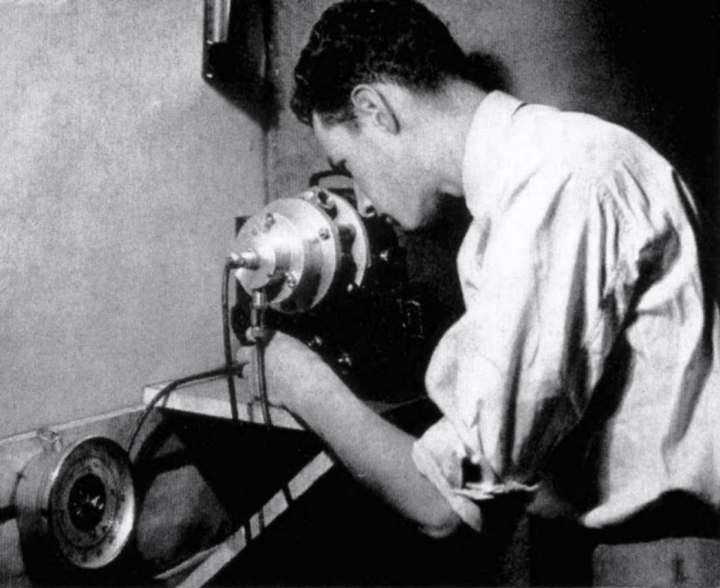
Micrometering Sound with Precision Pistonphone
