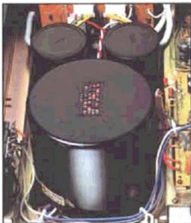
Huge toroidal core transformer of SX-1080.
