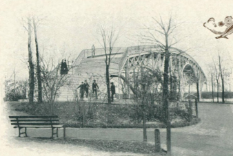
CANTILEVER BRIDGE OVER LAGOON, LINCOLN PARK, CHICAGO.
