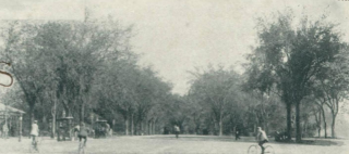
PLAZA ENTRANCE, CENTRAL PARK, NEW YORK.
